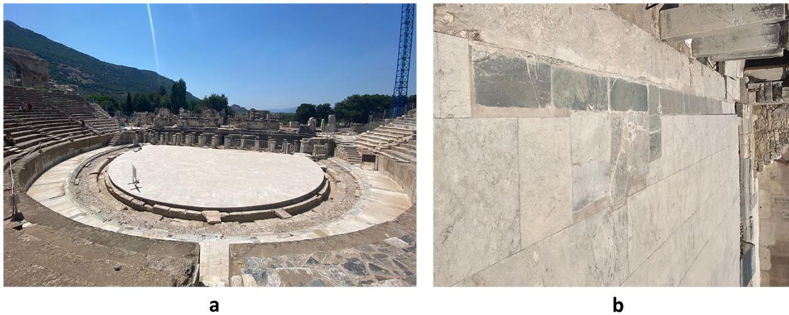
Figure 10. a. The orchestra after the completion of works between 2018-2021 (Yılmaz, 2021). b. Border mortar around the original paving stones (Yılmaz, 2019-2021)
