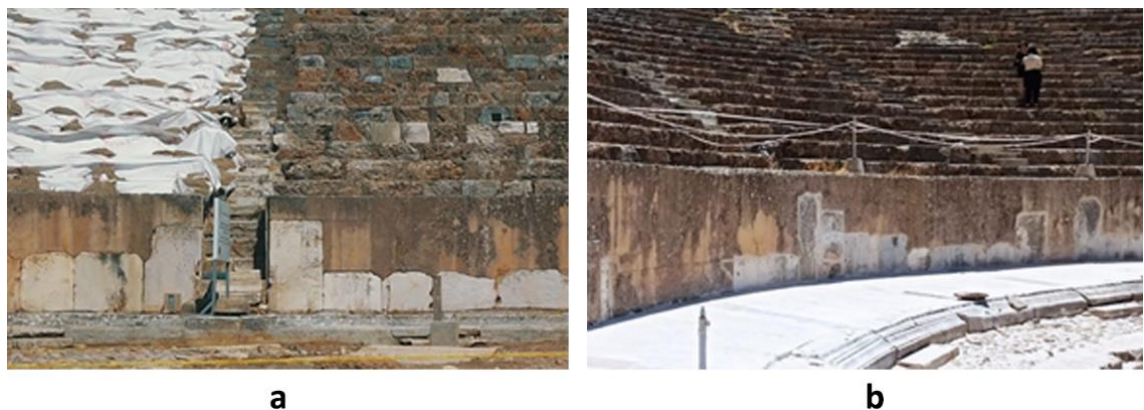
Figure 11. a. Restoration intervention on the orchestra retaining wall in the 70s (Republic of Türkiye Ministry of Culture and Tourism, 2021). b. The retaining wall and epicycle gap imitation with mortar after the works between 2018-2021 (Yılmaz, 2019-2021)
